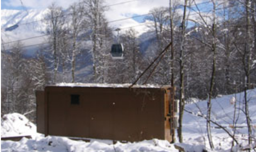
Thermally insulated containers protect the base stations in extreme conditions.
